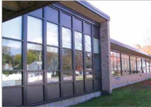
Ameresco installed new windows at the Reilly Elementary School.
