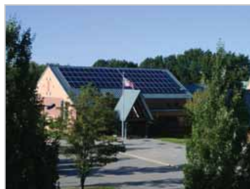
The Butler School with the solar photovoltaic (PV) array installed on the rooftop.
